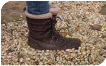
Too much aggregate
